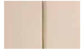
Hygiene Jointer (Knife edge embedded into silicon)
