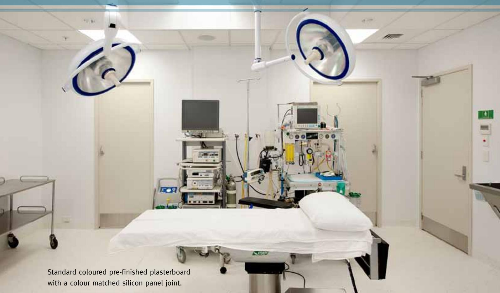
Standard coloured pre-finished plasterboard with a colour matched silicon panel joint.
