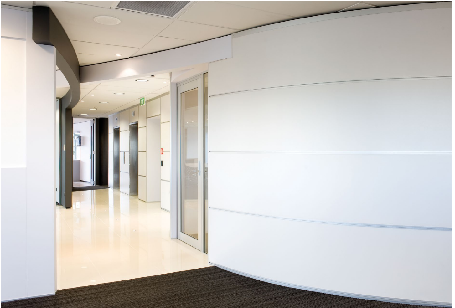
Reception - Arctic frost installed with negative detail jointer horizontally
